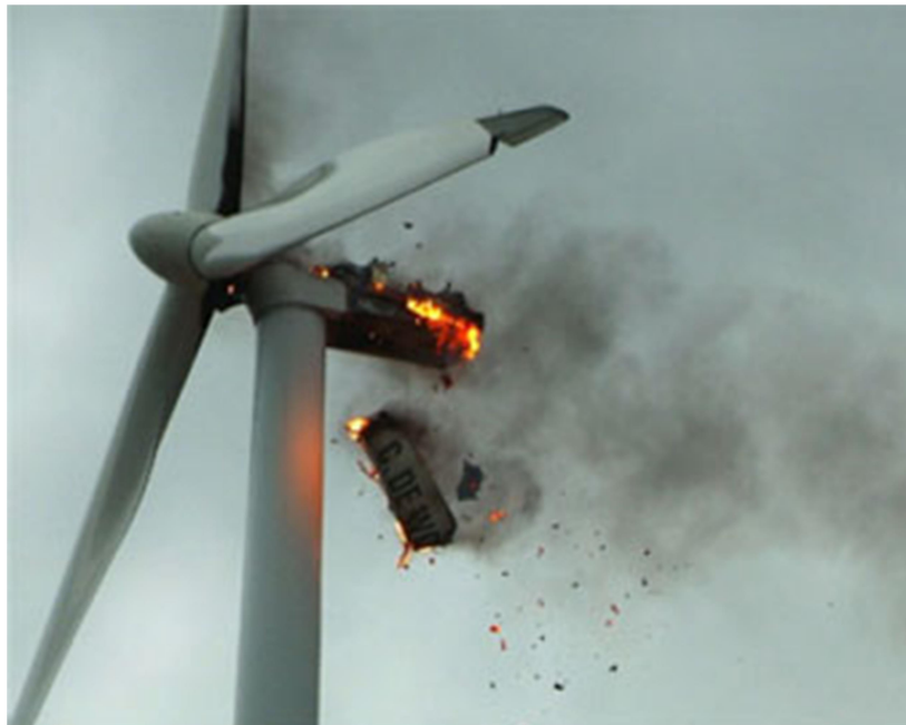
Figure 7.1 Fire in a wind-turbine generator.
