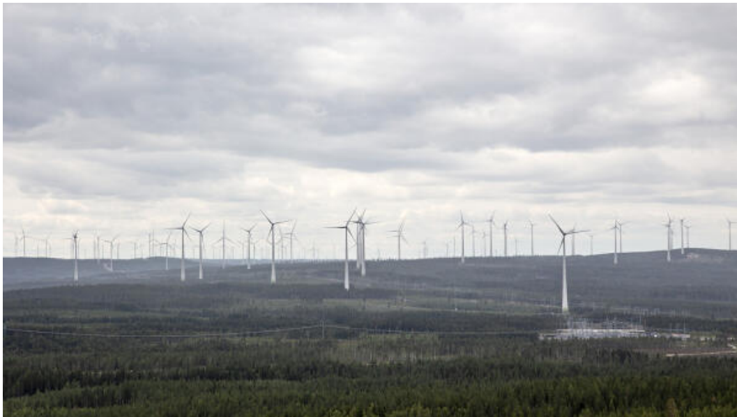
Figure 5.4 Wind power greatly affects local environment. The "turf" below the towers is a fully grown forest with 30 m high trees and one may just discern the power line among the tree tops in the foreground (Kalahatten at Piteå; archive photo by Helena Landstedt/TT).
