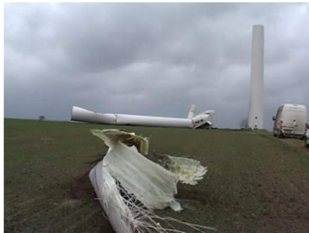
Figure 7.2 Collapsed wind-turbine tower.
